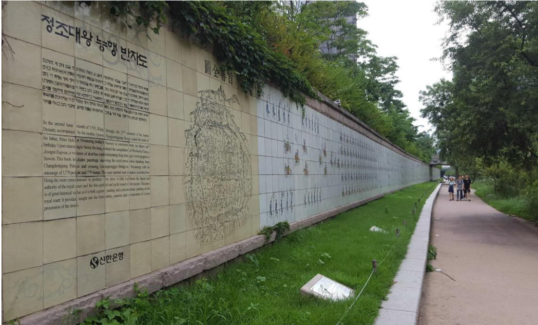
The beginning of the tile wall painting
